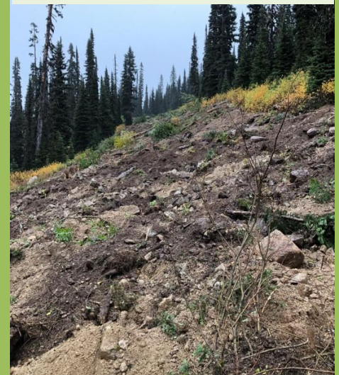
Example of road pullback and slope recontouring
